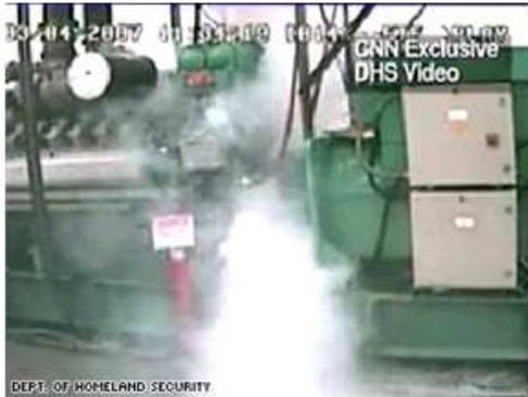
Experimental cyber-attack caused generator to self-destruct.
