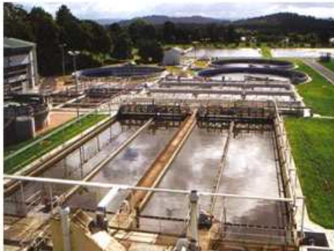
Sewage control system exploited by insider to cause sewage to flood the surroundings.
