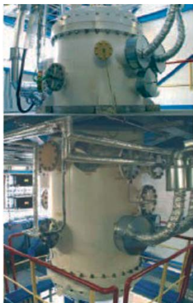
Figure 1: Pilot plant reactor DEMiSTM, DE-GUSSA, Hanau-Wolfgang
